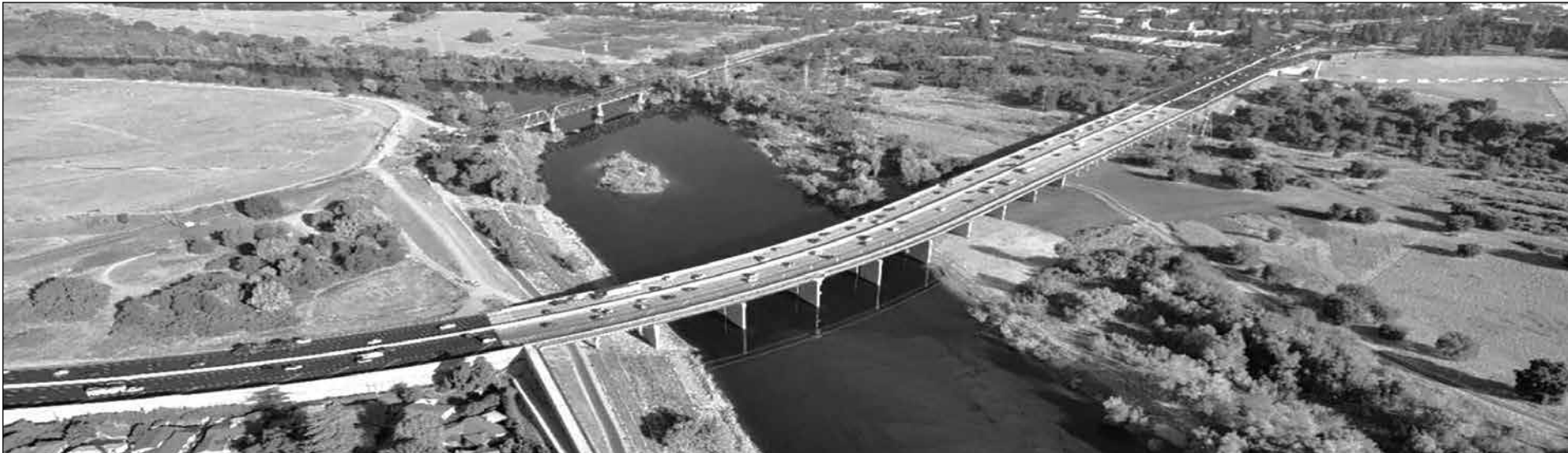
The improved bridge provides a multimodal connection between downtown and eastern Sacramento, linking residents and travelers to medical centers, employment opportunities and major activity hubs. Photo courtesy of California Department of Transportation
