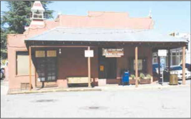
Old Town Auburn Post Office. Survived the fire of 1855.
