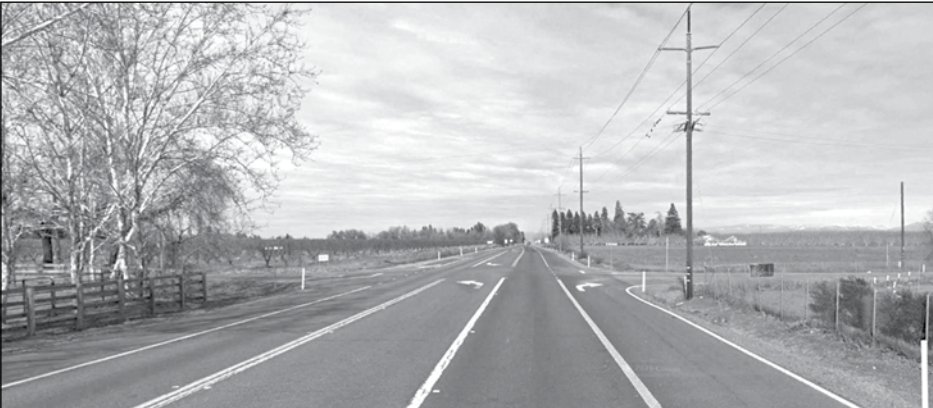
The intersection of Highway 99 and Rio Bonito Road currently requires motorists on Rio Bonito Road to stop while highway traffic continues without stopping. Caltrans is considering a traffic signal or roundabout to reduce collisions. Photo courtesy of Caltrans
