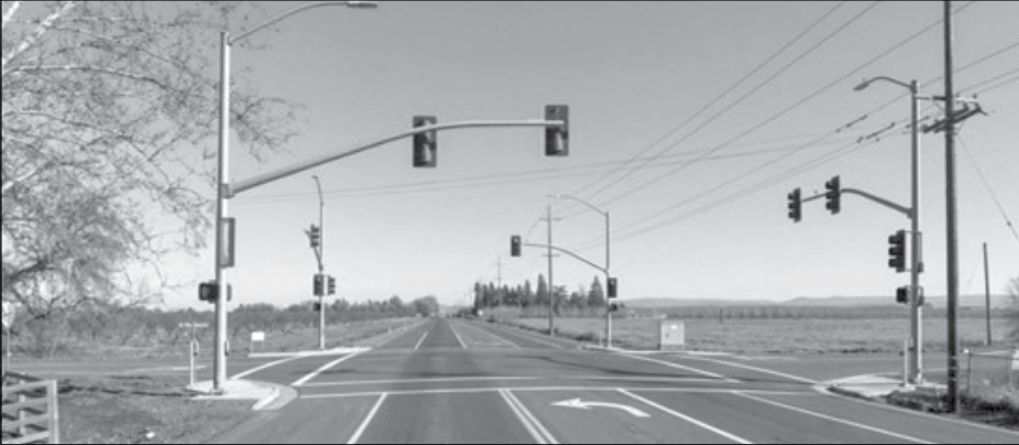
A traffic signal is one of two alternatives Caltrans is considering to improve safety at the intersection of Highway 99 and Rio Bonito Road east of Biggs. The project follows 15 broadside collisions recorded over five years. Photo courtesy of Caltrans
