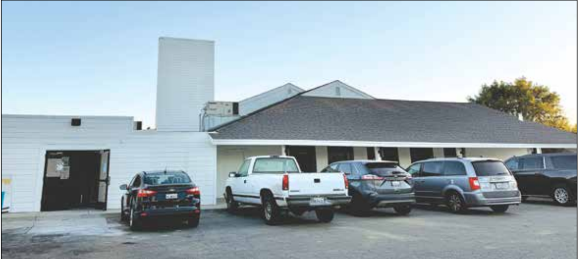
The newly renovated exterior of the Tri-Counties Community Center marks the completion of the first phase of improvements. The center will celebrate with a free community barbecue Nov. 7 while seeking support for its next phase of interior renovations.
