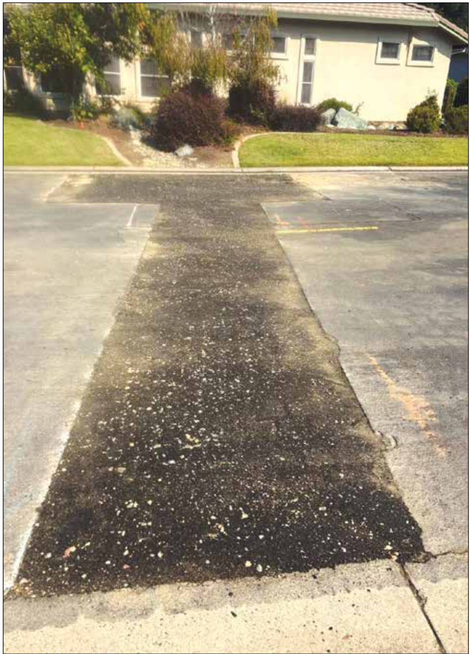
Photo shows the repair to a water service line on De La Cruz Drive. The final step will be restoring the asphalt. Photo courtesy of Rancho Murieta Community Services District
