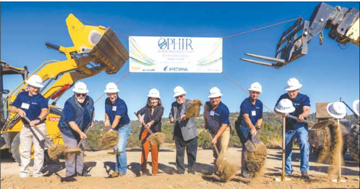
PCWA Board members and regional leaders ceremonially break ground on the Ophir Water Treatment Plant on Oct. 15, 2026. The $206 million facility will expand drinking water treatment capacity and strengthen water reliability in western Placer County. Photo courtesy of PCWA
