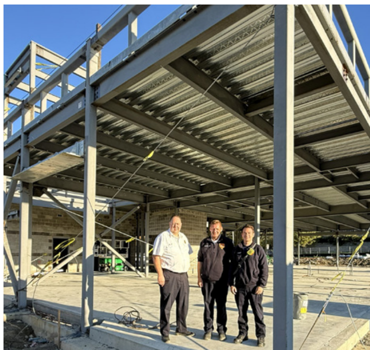
From left: Auburn Fire Chief Stephen Coleman, Deputy Chief Glenn Johnson, and Firefighter and President of IAFF Local 4157 Nick Fairbanks at the construction site. Photo by Walter Bird
