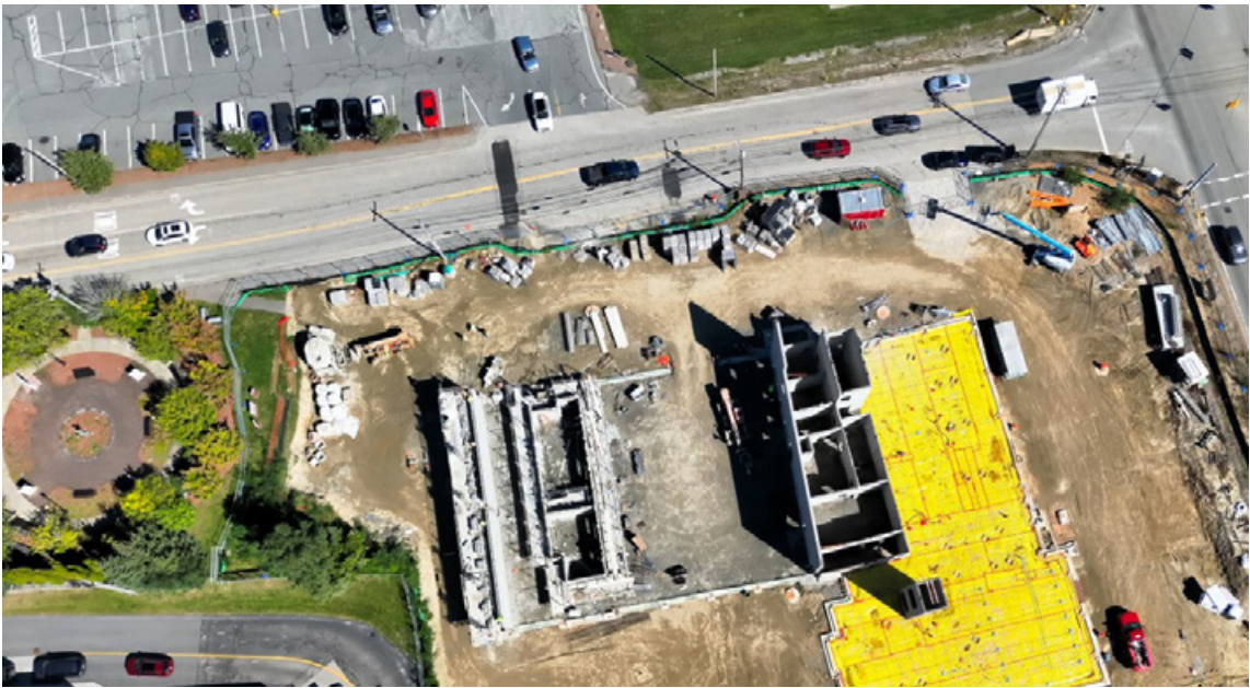
Aerial views of construction of the Auburn Fire Department's new headquarters at the site of the former Chuck's Steakhouse, 10 Prospect St. Courtesy of the Town of Auburn
