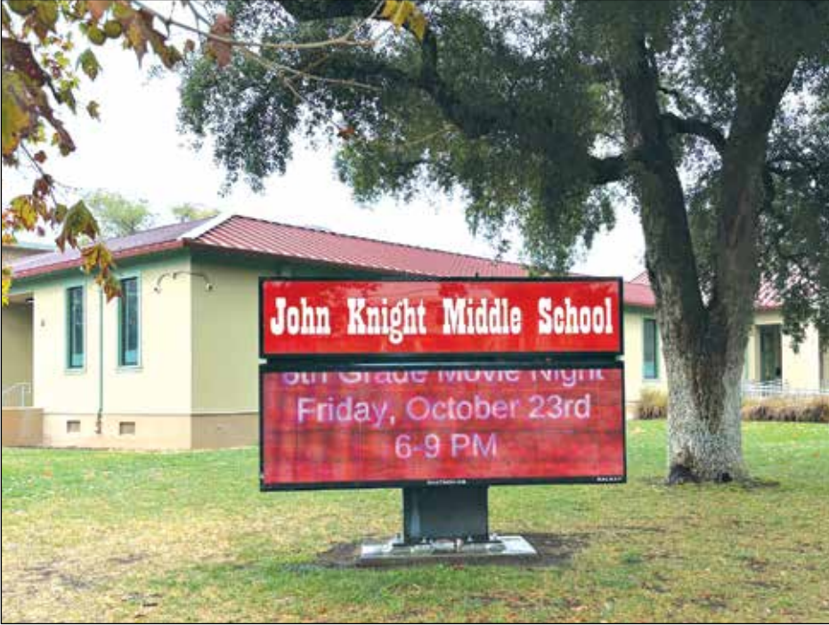
John Knight Middle School, on East A Street in Dixon, was renovated using funding from Measure Q, the 2016 bond issue
