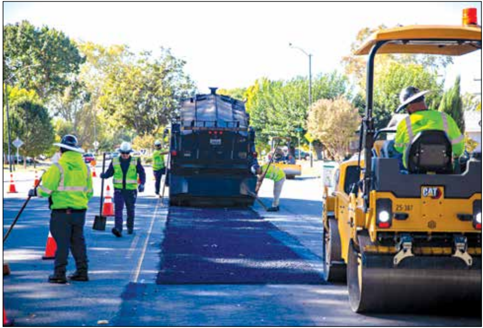
Repairs to Park Blvd will be completed in-house this fall, allowing surface treatment, striping and colored pavement work to begin in spring 2027. Photo courtesy of the City of West Sacramento
