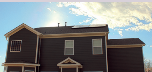
Scott Noel's home has a 2.616kW system comprised of eight SunPower 327W panels.
