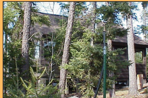
This cabin on Seagull Lake was protected by its working sprinkler system during the May 2007 wildfire. The cabins on both sides of this cabin did not have sprinkler systems and were destroyed in the fire.
