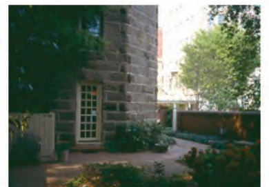
Tower courtyard entrance
