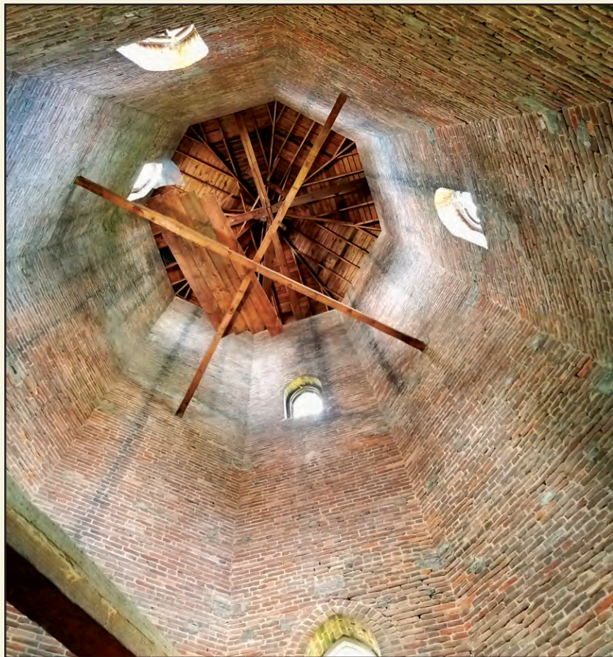
View of the tower roof from the fourth floor
