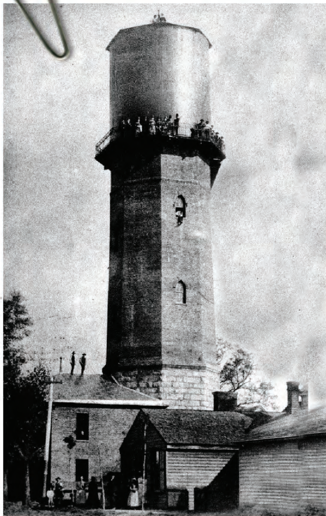
Tower with metal water tank, circa 1887
