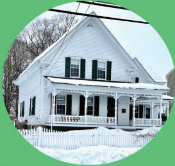
19 Church Street Franklin
