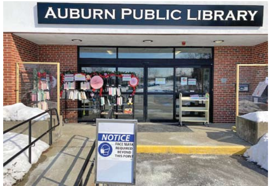
The entrance to the Auburn Public Library. As part of a $1 million redevelopment project in the town of Auburn, the library will get a sunroom off the back of the building, and a connection to Goddard Park by way of a pedestrian bridge.
