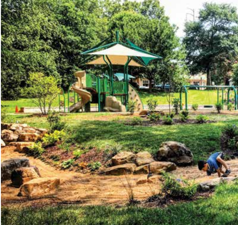
In Ormond-Grant Park, a green infrastructure amenity helps to prevent flooding of the park. (Photo: Michael Halicki)
