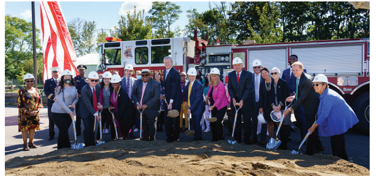
Groundbreaking was held on September 29 for the MassBay Center for Health Sciences, Early Childhood, and Human Services. Photo courtesy of MassBay Community College.
