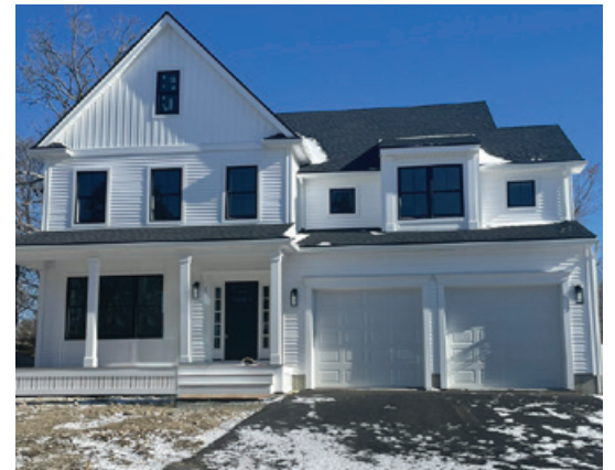
UNDER CONTRACT 13 HARWOOD RD, NATICK
