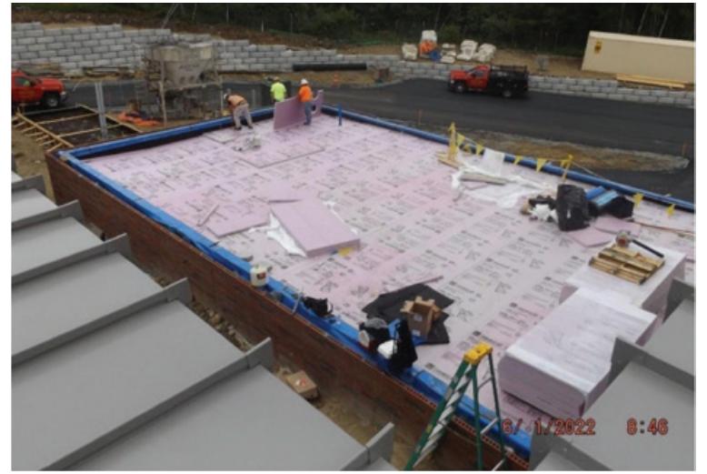
The Progress of the lower green roof.
