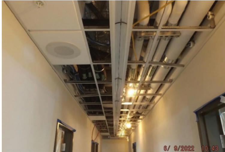
The Progress of the third floor finishes—paint and ceiling grid.
