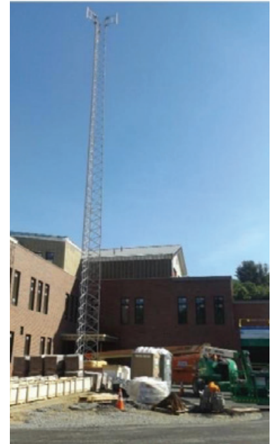
Installation of the communications tower.
