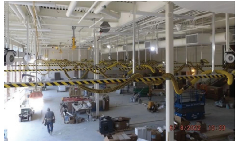
The Progress of the apparatus bay.
