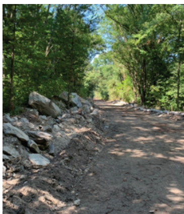
Boulders, trees, brush and debris removed from the trail to make it clear, accessible and safe.
