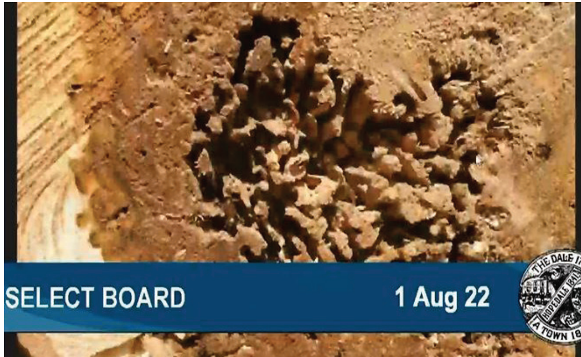
Inside of tree that was removed from 61 Bancroft Park due to decay. Source: Hopedale Select Board, Aug. 1, 2022.
